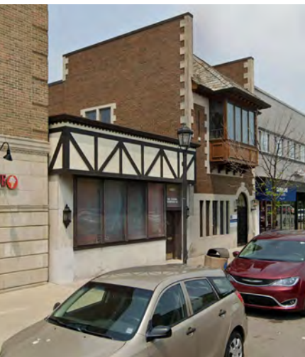
Current condition of 16825-16835 Kercheval
